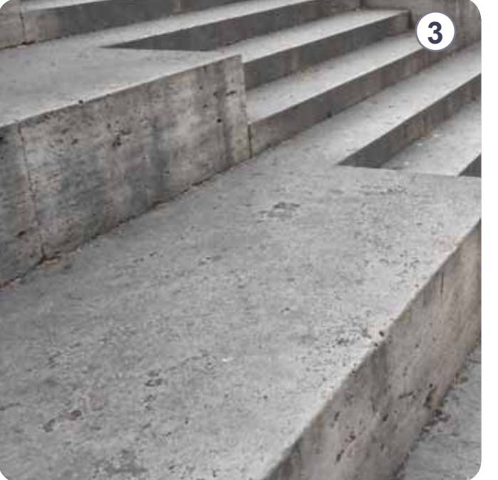
Concrete bleachers with inbuilt steps
